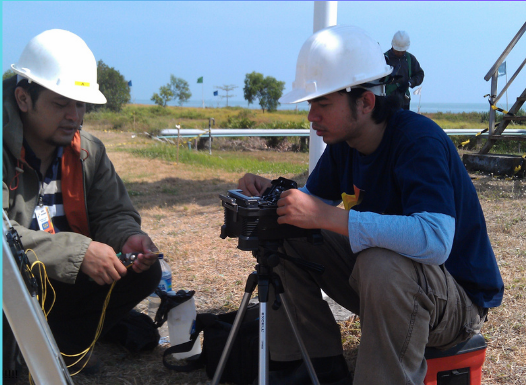
Fiber Optic Instalation Pertamina Balongan
