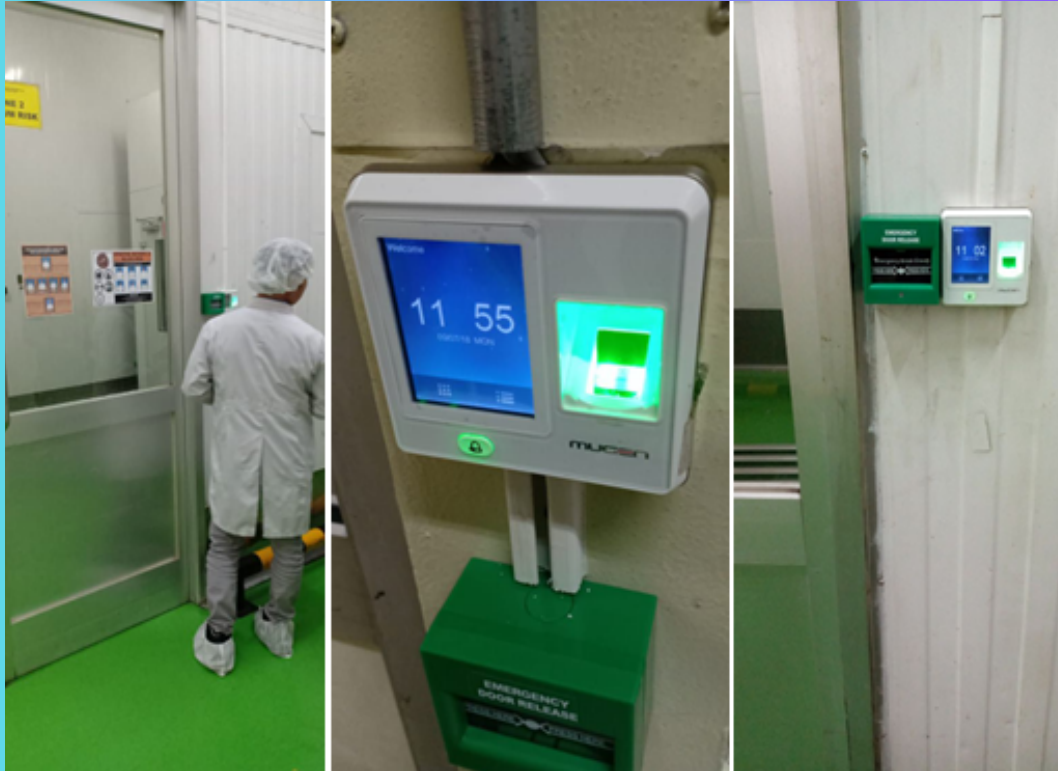
Access Door Instalation PT Ultrajaya
