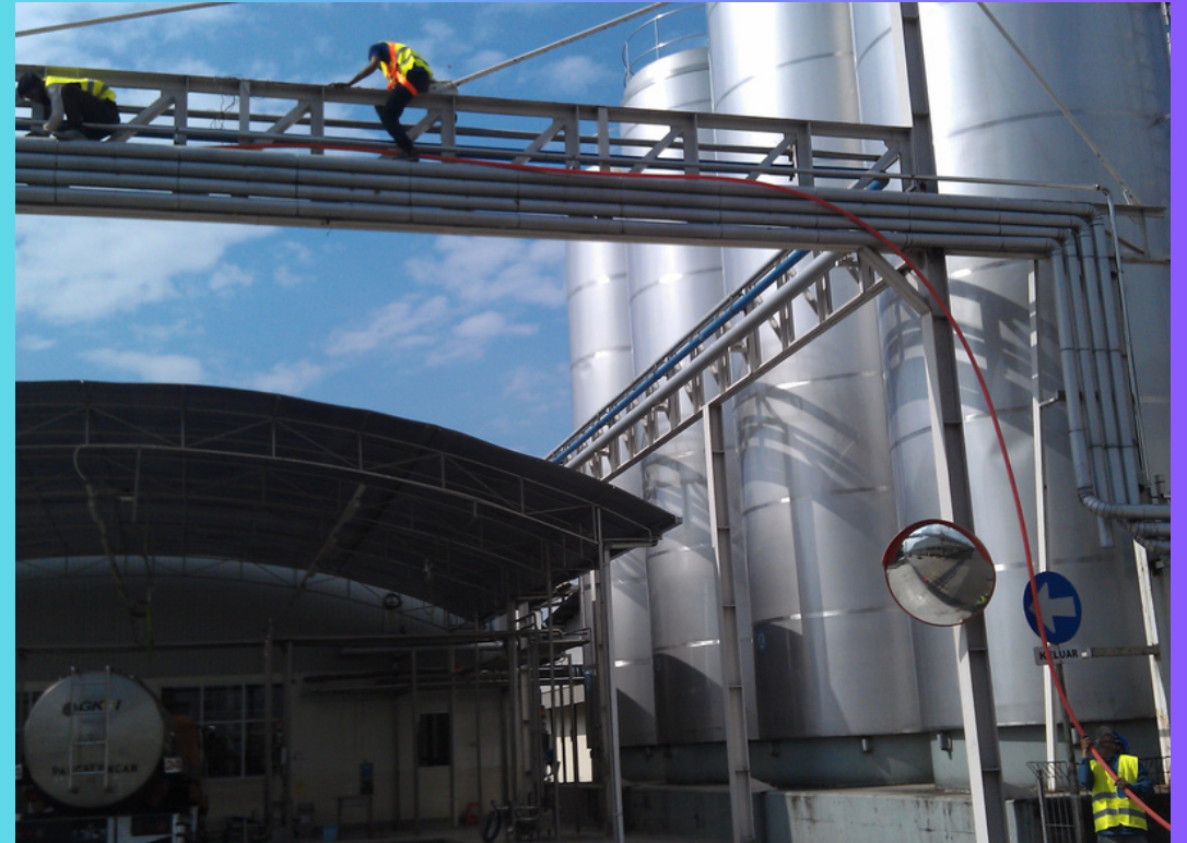
Fiber Optic Instalation PT Ultrajaya
